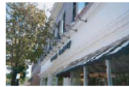
Lighting should be designed as an architectural element and integrated with the building design.
