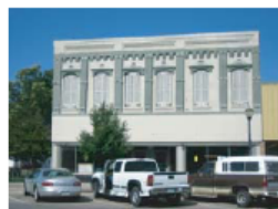
An example of operable shutters facing the street.
