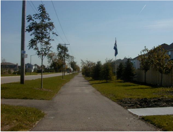
Example of a Shared-use Path in Plainfield
