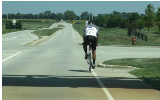
Curbs protruding into the shoulder push bicyclists into the travel lane (Shown here at Ridge Road and Grand Park Boulevard)
