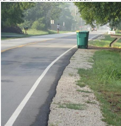
Figure 4.5 Paving the entire shoulder on this segment of Plainfield- Naperville Rd will encourage more bicycle travel Source: www.communityremarks.com Heath
