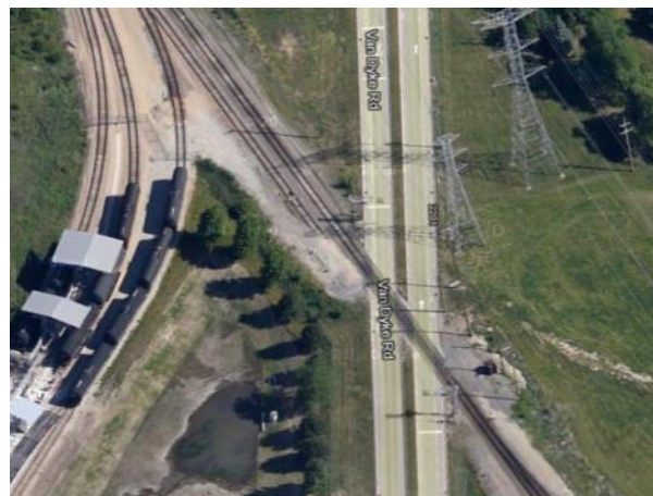
Figure 4.12 The angular railroad crossing along Van Dyke Road
