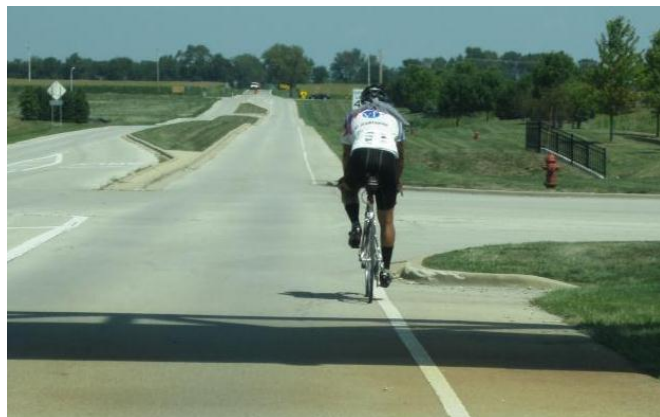
Figure 4.6 Curbs protruding into the shoulder push bicyclists into the travel lane (Shown here at Ridge Road and Grand Park Boulevard) Source: www.communityremarks.com Heath
