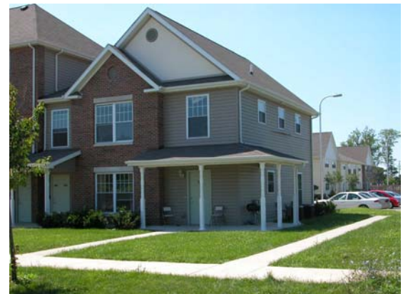
One key to obtaining urban development is reducing developer risk.
