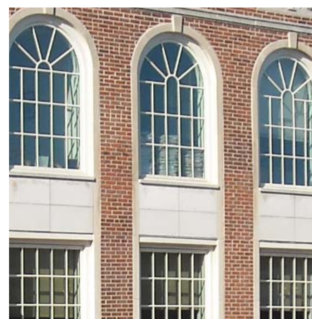
Arched fenestrations with intricate window paneling adds distinction to this two story brick building.
