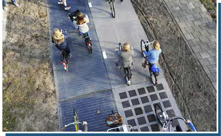
Dutch bike trails have a solar powered trail surface which produces solar energy. Located near ComEd power lines in Northfield, the community may consider similar technology to acknowledge the lines and serve as a green power source.
