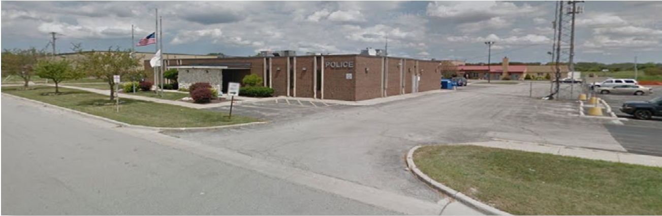
Existing building and site of the Sauk Village Police Department
