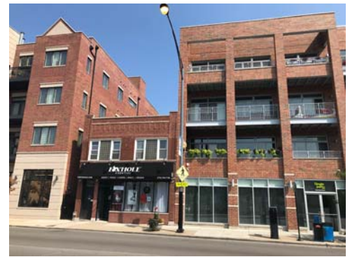
C Mixed-Use Buildings between Artesian and Campbell
