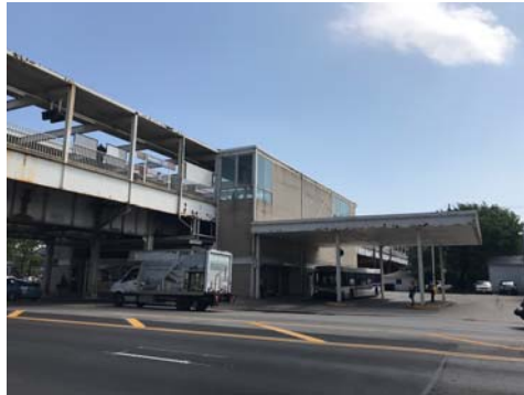
B Western Ave Brown Line CTA Station
