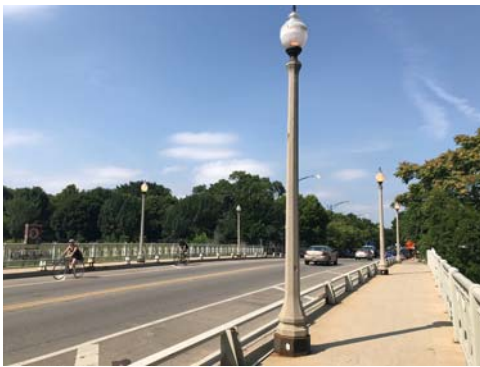
A North Branch Chicago River Bridge
