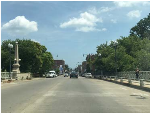
A North Branch Chicago River Bridge
