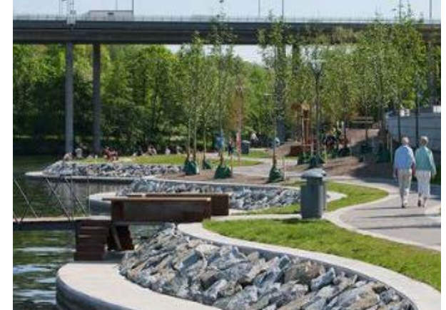
Concrete river edge walk with rock riprap. This was a popular idea to include in the park.
