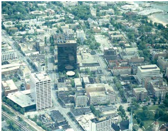
State National Bank Plaza (dark tower) and the American Hospitals Supply Corporation Headquarters (white tower)
