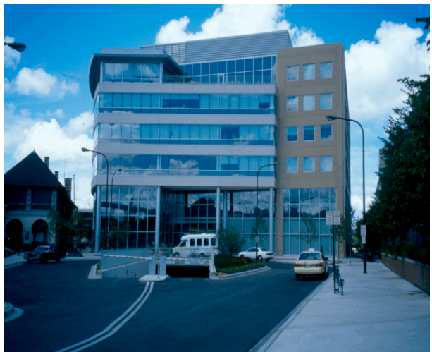
909 Davis Street: Phase 2
