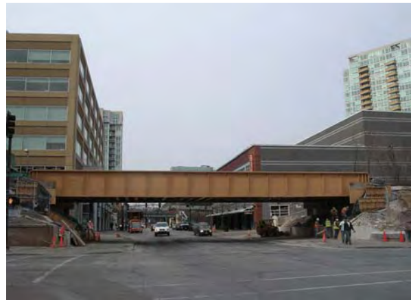
New Church Street Viaduct
