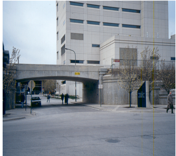
Clark Street Viaduct
