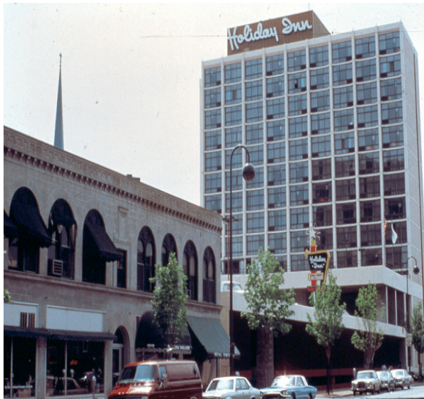
Holiday Inn Hotel & Parking Garage
