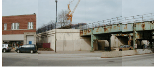
Davis Street With Unused Union Pacific Viaduct
