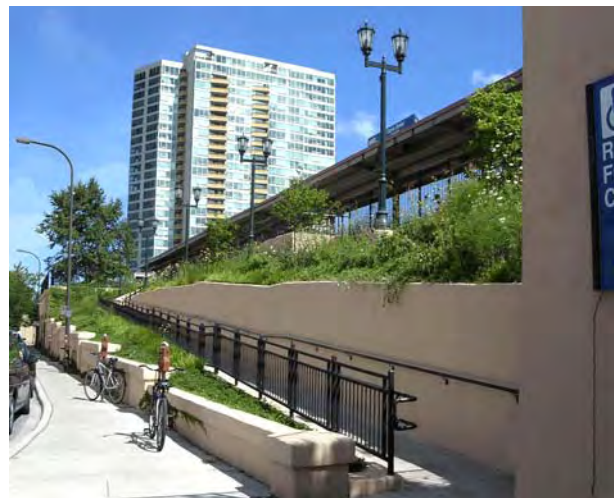
Metra Station ADA Ramps
