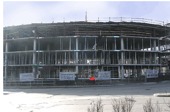
Grand Bend @ Green Bay Under Construction
