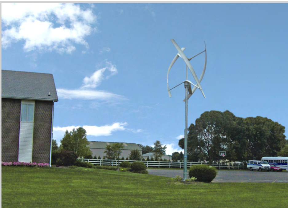
NEWLY INSTALLED VERTICAL ACCESS WIND TURBINE AT VALLEY BAPTIST CHURCH IN KENDALL COUNTY
