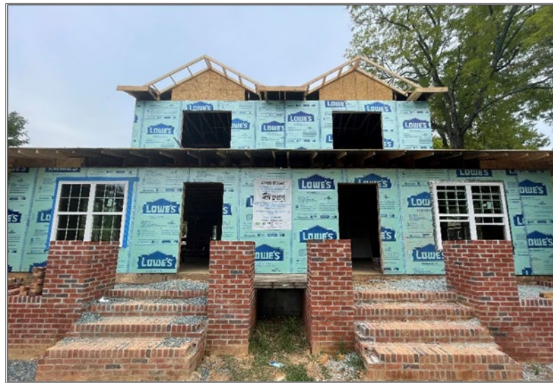
Habitat for Humanity homes under construction on Cobb Street
