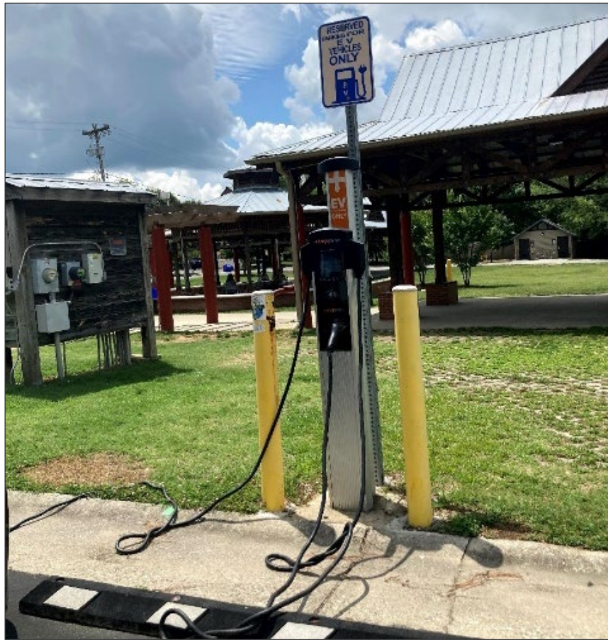
Electric vehicle charging station in Carrboro.
