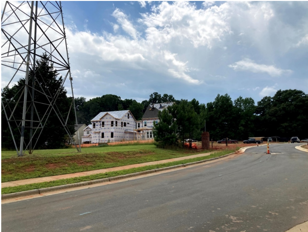
New construction of housing often includes energy efficiency updates.
