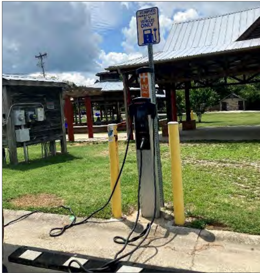
Electric vehicle charging station in Carrboro.
