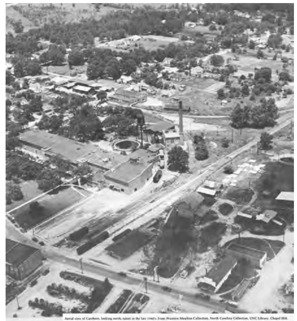
Aerial view of Carrboro, looking north, taken in the late 1940s. From Phyllis Meeker Collection, North Carolina Collection, UNC Library, Chapel Hill.
