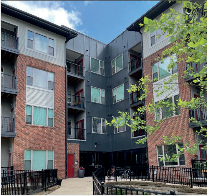
Shelton Station includes 20% affordable housing units and is located a short walk to Carr Mill and Downtown Carrboro.
