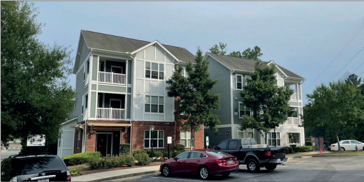
The Landings at Winmore is a 58-unit Community Home Trust affordable rental development in Carrboro
