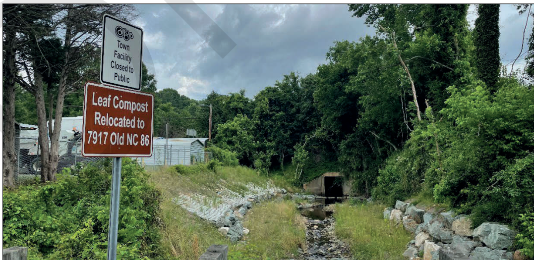
One of the ways Carrboro can continue improving water quality is by pursuing stream restoration, enhancing stormwater runoff management projects.
