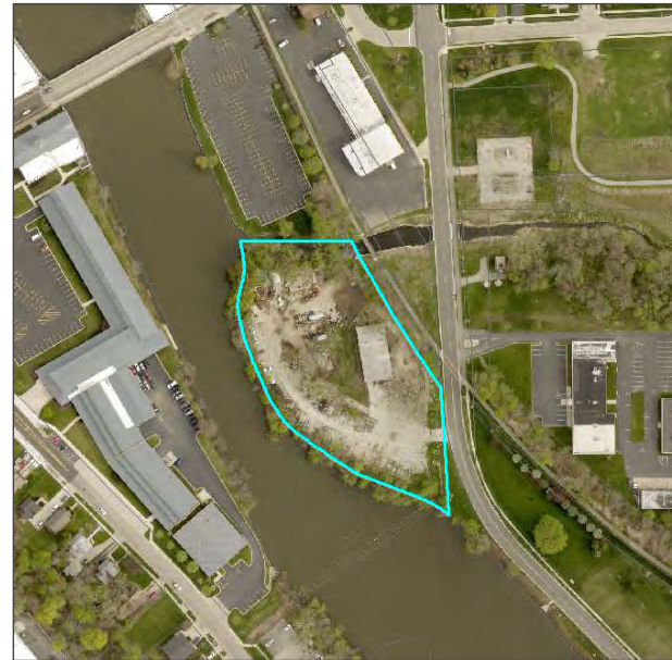
M & M Patio Stone Site, Aerial
