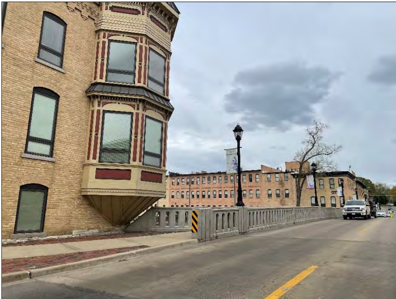
Main Street Bridge Connects Old Town Former Mill Buildings
