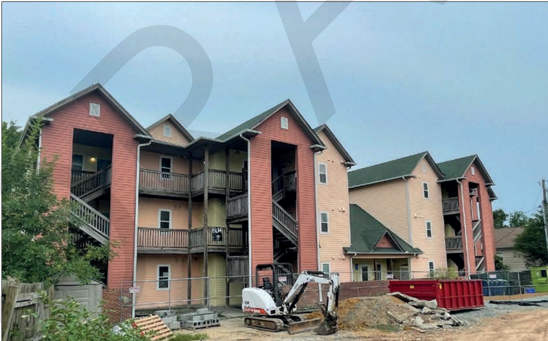
A new clubhouse for Club Nova is being built in front of affordable housing along Main Street in Downtown
