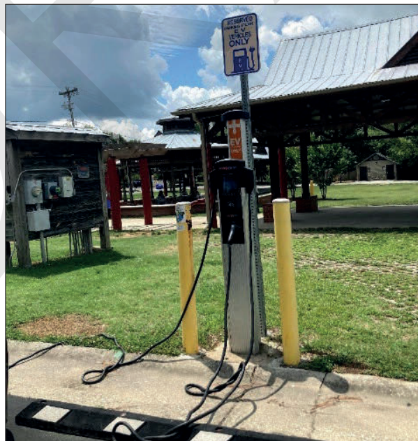
Electric vehicle charging station in Carrboro.
