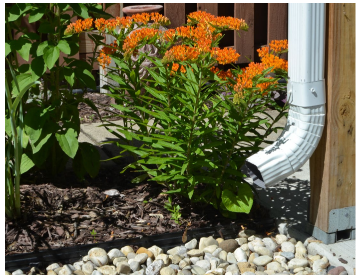
Impervious removal and disconnection
