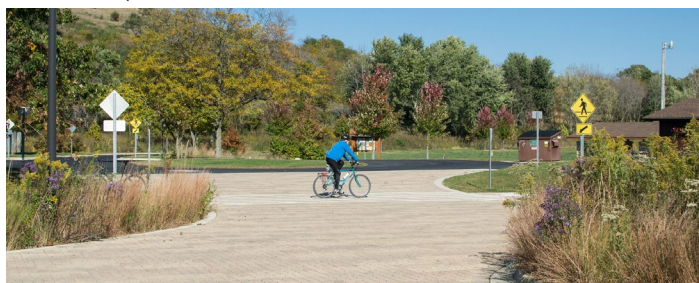
Permeable pavement & bioretention bump-outs
