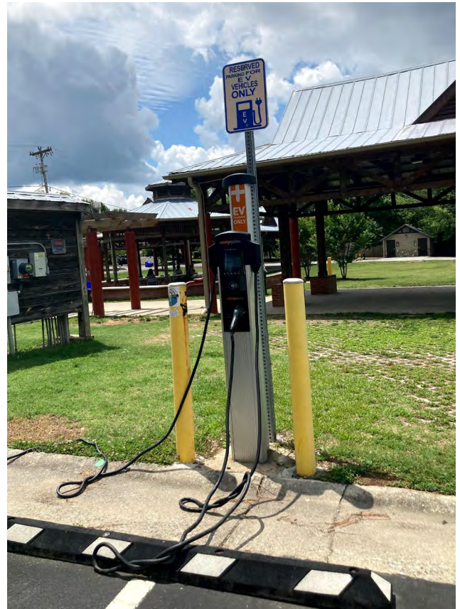
▲ Electric vehicle charging station at Town Commons
