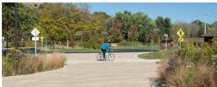
Permeable pavement & bioretention bump-outs
