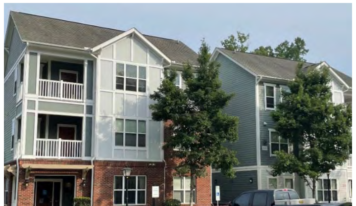
▲ The Landings at Winmore is a 58-unit Community Home Trust affordable rental development in Carrboro
