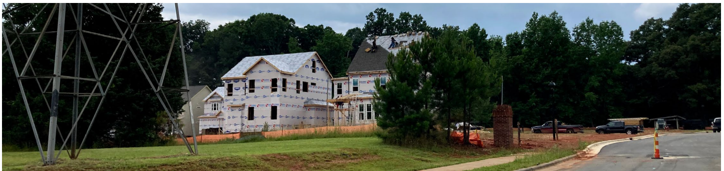
▲ New construction of housing often includes energy efficiency updates.
