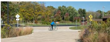
Permeable pavement & bioretention bump-outs
