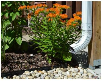
Impervious removal and disconnection
